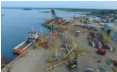
Petromar Fabrication Yard (Soyo e Ambriz)
