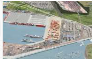
Dande Oceanic Terminal
